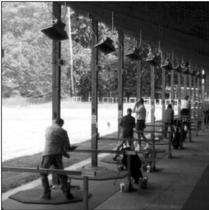
Golf Driving Range Installation with heaters mounted at nine feet and capable of raising the target area (you) by 20 degrees F.
