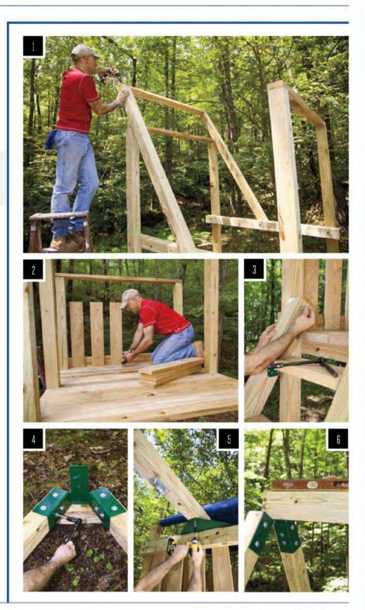
lag-screw it to the post ends [1]. Stand the canopy posts upright and use a 4-foot level to ensure they're plumb, then tighten the nuts on the bolts.
